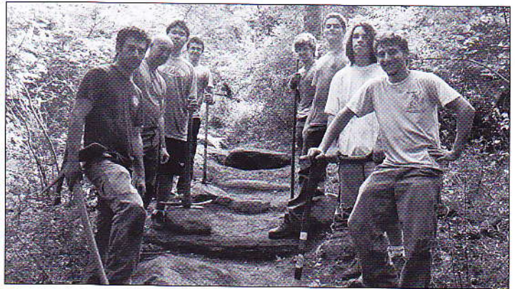
Ramapo Reservation Trail Work
